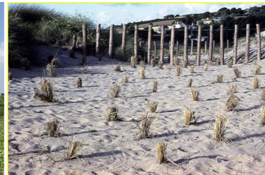
Protecting sandy edges with ground cover and temporary fence
