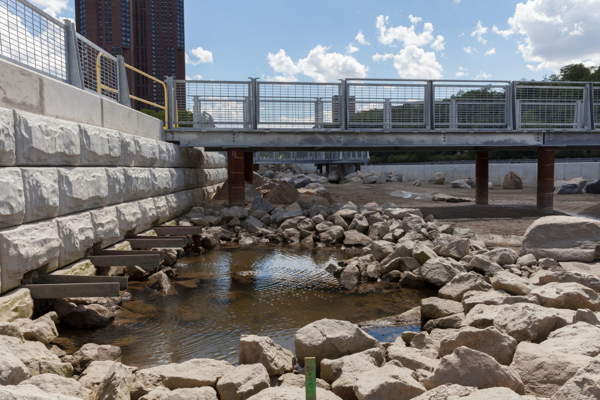
9. This photo taken during construction demonstrates how collected storm water from the upland is captured and filtered through the tidal marshes before entering the Harlem River.
