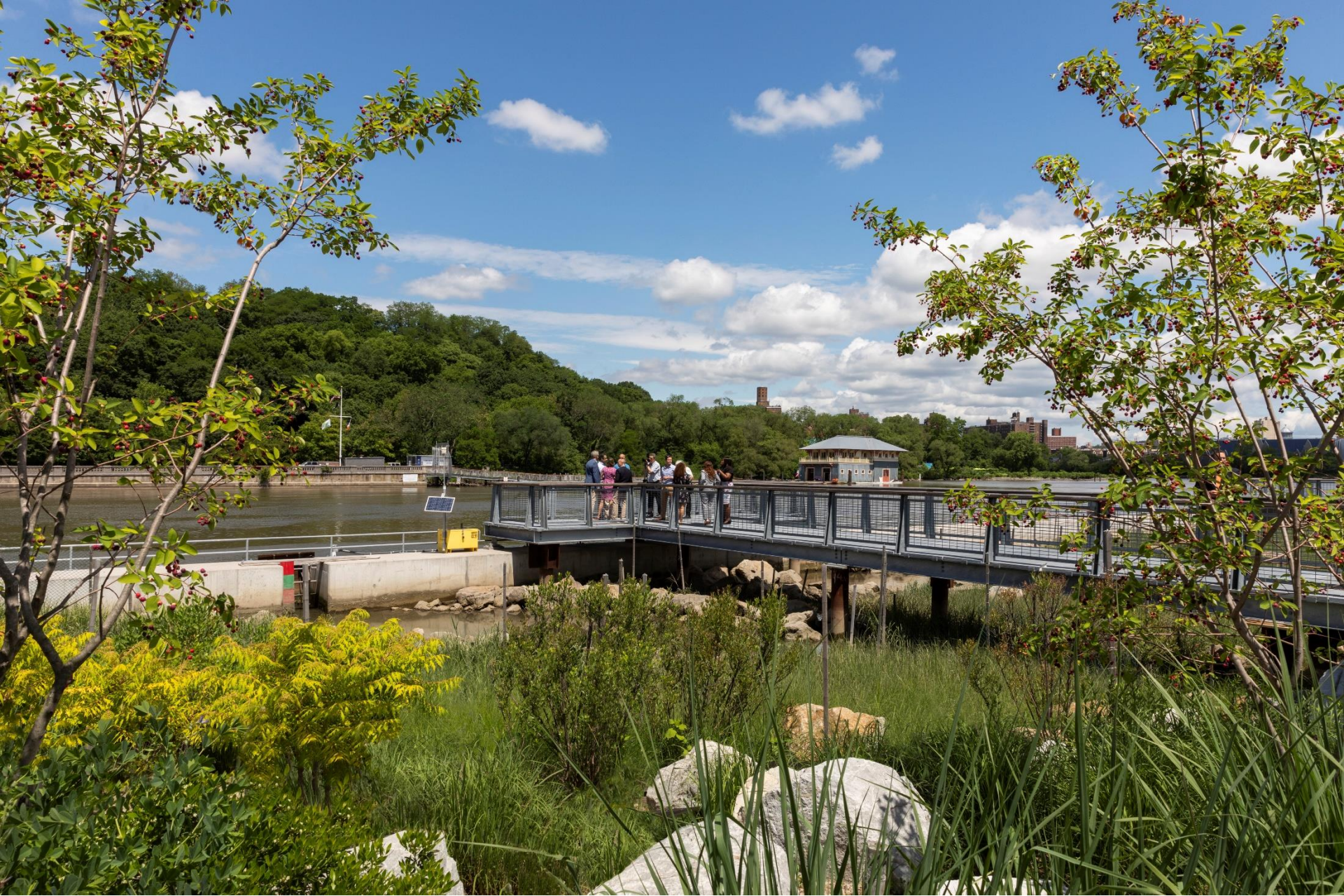
14. Located at either end of the marsh, the scrub-shrub showcases a variety of plant species that serve different ecological functions that include food sources for birds and pollinators. Plant heights and elevations within these areas were closely coordinated to frame views of the marsh and the river.
