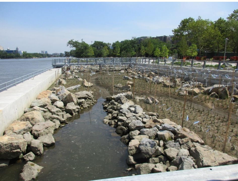
11. The construction process can be seen here after the boulder installation at mean and high tide, and immediately after initial plant installation.
